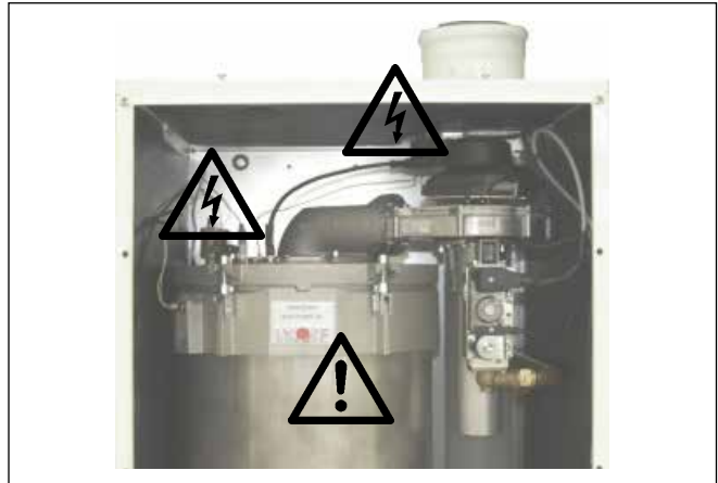
Figure: Ignition transformer, ignition electrode, heat exchanger
